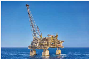
Wheatstone LNG Project, Australia Source: Chevron Australia
